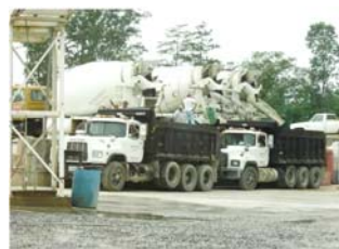
Dry-Batch Concrete Plant
